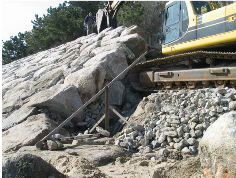
Figure 1. Representative photograph of the reconstructed revetment.
